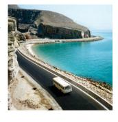
and steep face rugged mountains. The project road was designed with some of its sections going directly along the sea while the other sections were constructed over rugged mountains with cliff-like ridges. The embankments on the coastal side were provided with specifically designed revetment stone protection layer against sea wave/tidal action.
