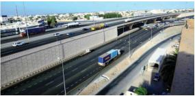
taxi stands and bus bays. The project scope also comprised expropriation of properties, relocation/protection of services, road lighting works and traffic signals. Completion of this 8km project has mitigated traffic congestions in the Sohar area and eased the movement of traffic approaching/passing through the city
