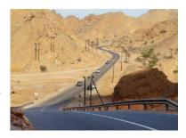
the road posed a big challenge to NESPAK due to the mountainous terrain and several Wadis along the alignment. The 7metres wide road having paved shoulders on both sides serves as a vital route for interregional trade, commerce and tourism in the Sultanate of Oman. The cross drainage structures include bridges, pipe & box culverts and Irish crossings.
