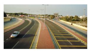
The dualisation of 24 km long Mulladah Al-Hazm Road project involved the construction of an additional carriageway, the rehabilitation of the existing road, three roundabouts, three underpasses, streetlighting systems and service roads. The road was dualised up to Rustaq connecting it further to the Ad Dhahira Region through a single carriageway. The Government of Oman has highly appreciated the quality of work carried out by NESPAK.
