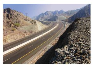
The 80 km long carriageway is an important link between the Sultanate of Oman and the United Arab Emirates (UAE) and carries inter-regional and cross-border traffic from Sohar Port to Buraimi and Al-Ain City and other UAE states. The project comprised the construction of an additional carriageway, 18 new bridges, two underpasses, an interchange to connect the new seaport, service roads and cross drainage
