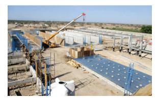
The project encompasses 67970m Sewerage Network, 8000m force main, 2000 house connections, Sewage Pump Station and a 4000 m³/day capacity Sewage Treatment Plant with extended aeration activated sludge process in the Wilayat (town) of Al-Musannah.
